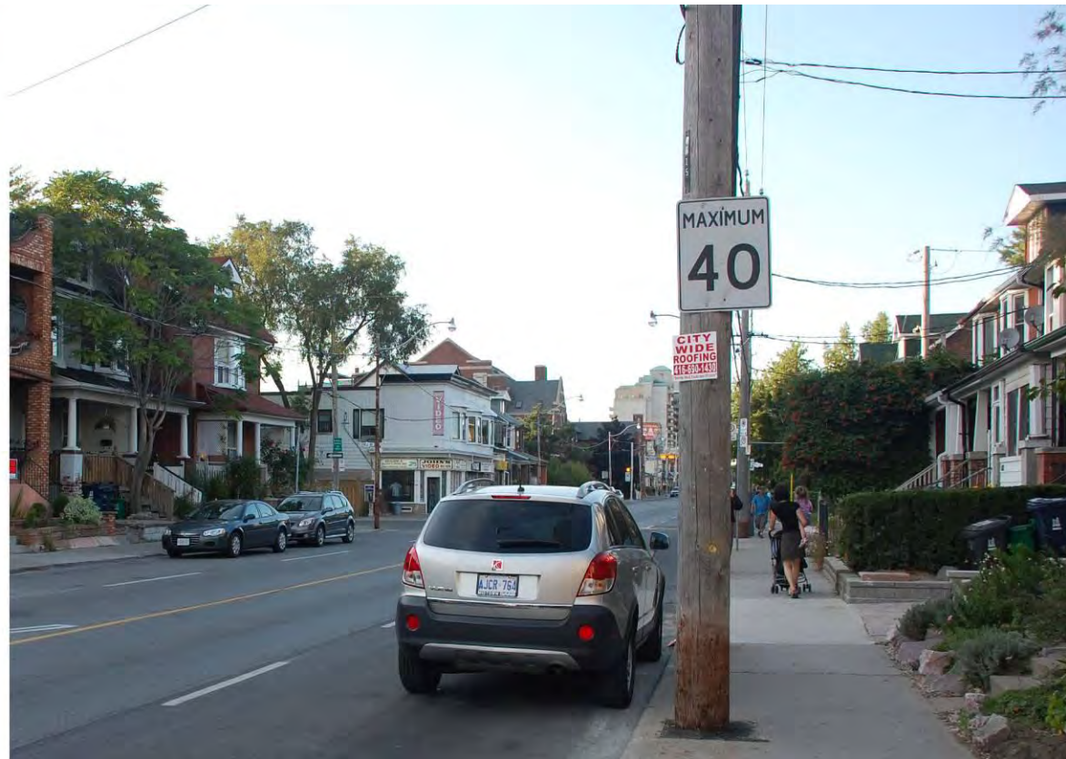
Wood poles – Pape Avenue
