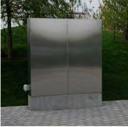
BIA Metering Cabinet / BIA Panel (Sugar Beach) 1.2m x 1.5m x 0.6m exterior dimension 3m clear in front required *Finish shown is not typical
