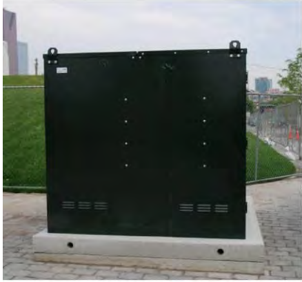
TX Pad-mounted Transformer (Sugar Beach) 2m x 2m exterior dimension 7m x 4m clear required
