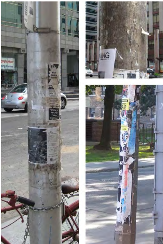
Adhesive residue on metal pole
