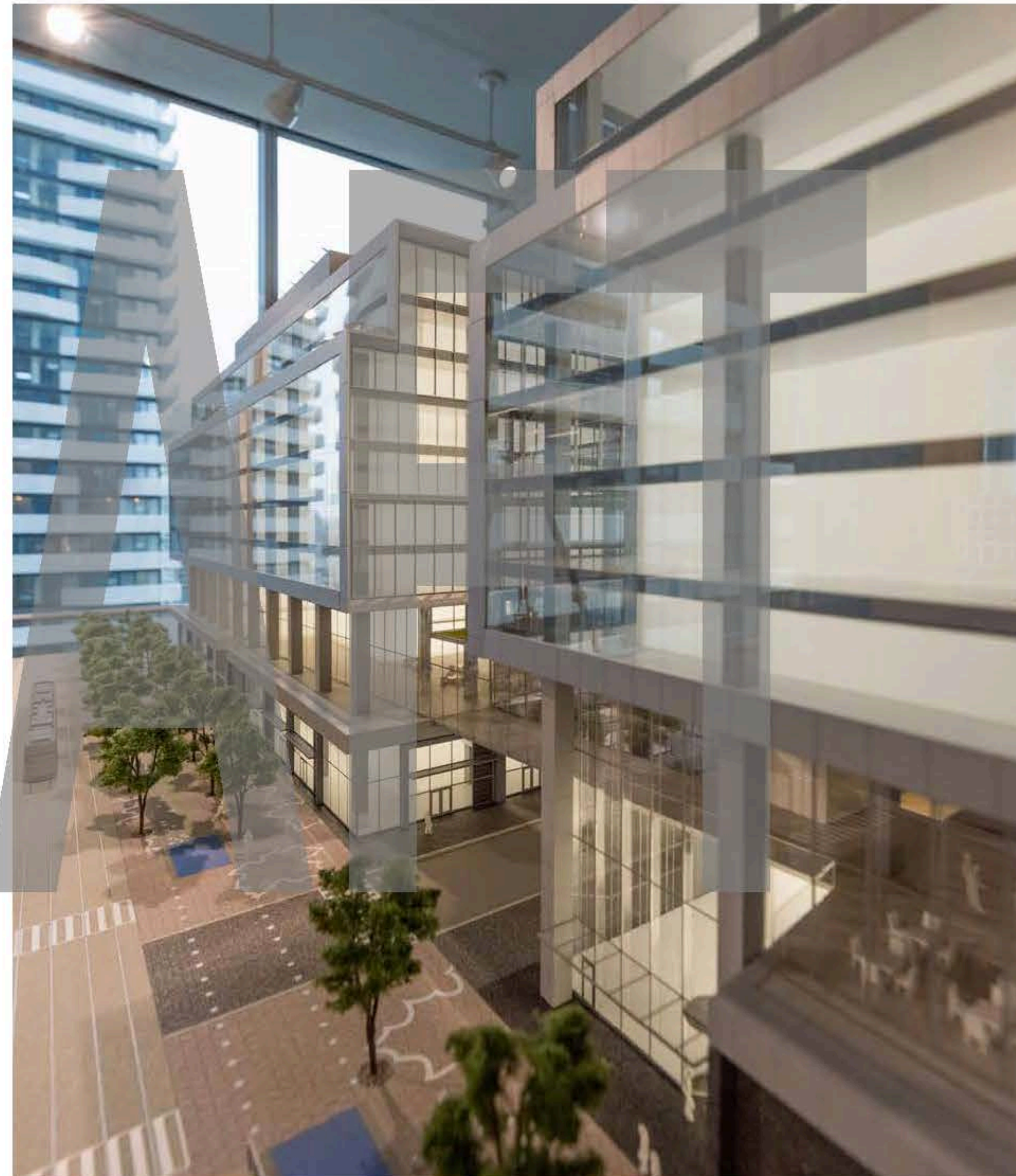
Detailed View - North Facade Along Queens Quay East
