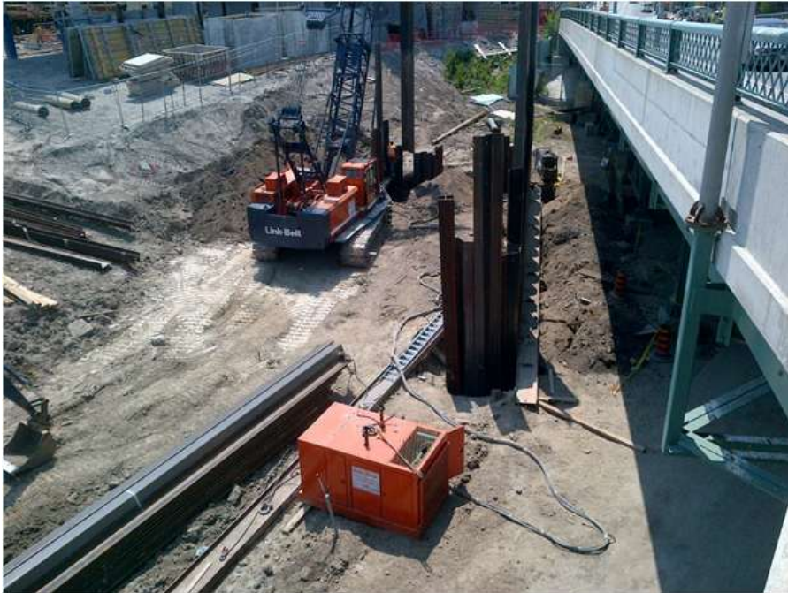
Sheet Piling for 1650 Back Flow Preventer under Queen Street Bridge
