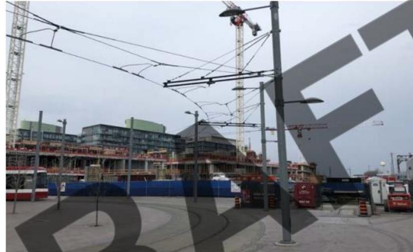
2. Southwest corner on Cherry St. Corner looking northeast
