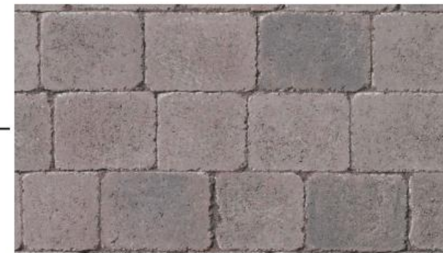
A band of concrete pavers (paleo-tech /Waterfront Toronto Standard) is used to delineate the large banding field pattern within the public open space.
