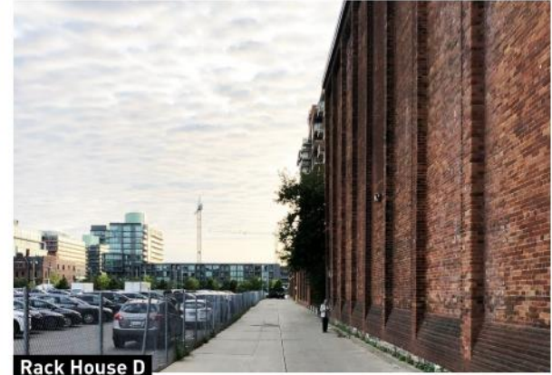
Rack House D
