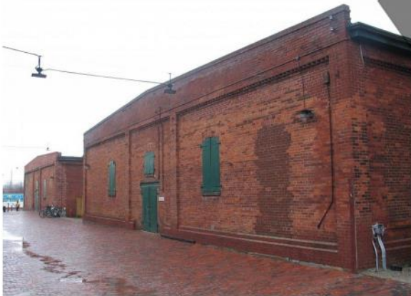
BASE / TOP - INVERTED RACK HOUSE
