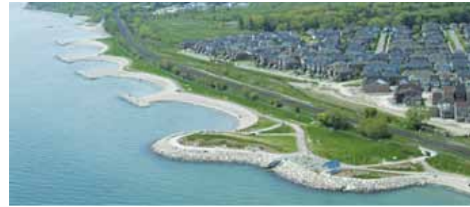
Port Union Waterfront Park – The project includes improved recreational access to the waterfront, cobblestone beaches, shoreline protection, 3.6 kilometres of waterfront trail, pedestrian lookouts and connections, and improvements to aquatic and terrestrial habitats.
