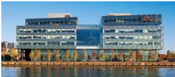
All buildings on Toronto's waterfront, like Corus Quay, will be energy-efficient and LEED Gold certified.
