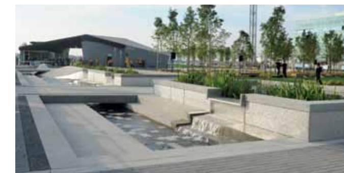
More than just a beautiful public space, Sherbourne Common is also the first park in Canada to integrate a stormwater treatment facility into its design. Stormwater is treated in a UV facility located in the basement of the park's pavilion, then released from three dramatic art features into the park's urban river and flows into Lake Ontario.
