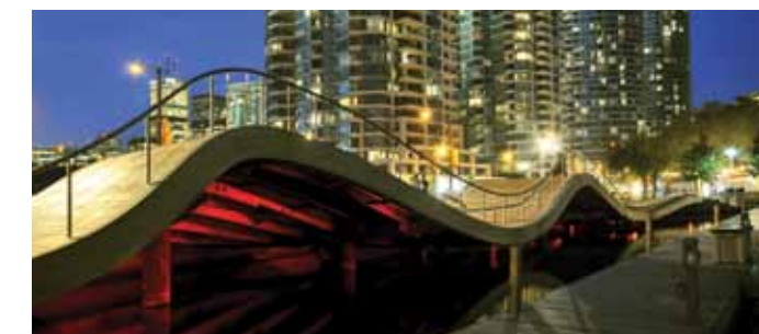
Above: Simcoe WaveDeck features curves that soar as high as 2.6 metres above the lake, and it is a popular attraction at all times of day. Large Image: Queens Quay looking east at the Simcoe WaveDeck.
