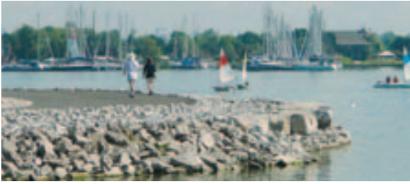
Mimico Waterfront Park – Restoration and shoreline enhancements to terrestrial and aquatic habitats form key elements of the park. It features a new section of the multi-use waterfront trail, a breakwater island to protect the new aquatic plantings, and new sand dunes and cobblestone beaches.
