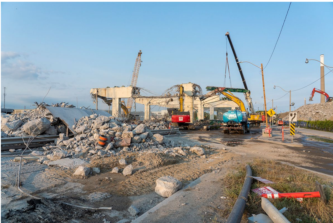
Above: Looking west at Don Roadway, you can see the last remaining steel bent. This bent will be removed as soon as the traffic lights are relocated to a new structure.
