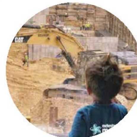
Water tunnel construction viewing
