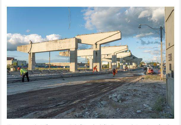
Above: Crews made significant progress in the first weekend of work to remove the Logan Ramps from the Gardiner to Lake Shore. Looking west from Lake Shore, you can see where the deck has been removed.
