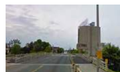
KEATING CHANNEL BRIDGE
