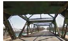
SHIP CHANNEL BRIDGE
