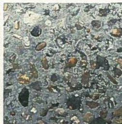
Concrete with 20-50mm recycled aggregates + exposed aggregate finish
