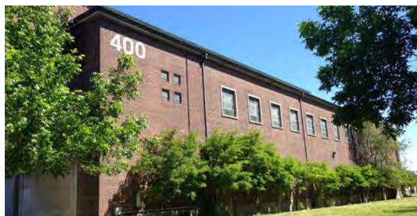
400 Commissioners Street Transfer Station
