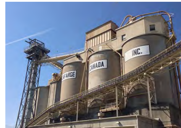
Lafarge Silos on Polson Quay
