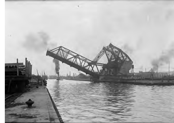
1920s Cherry Street Bridge (North Bascule) (Source: City of Toronto Archives)
