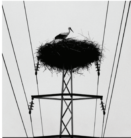
Stork nest on a transmission tower
