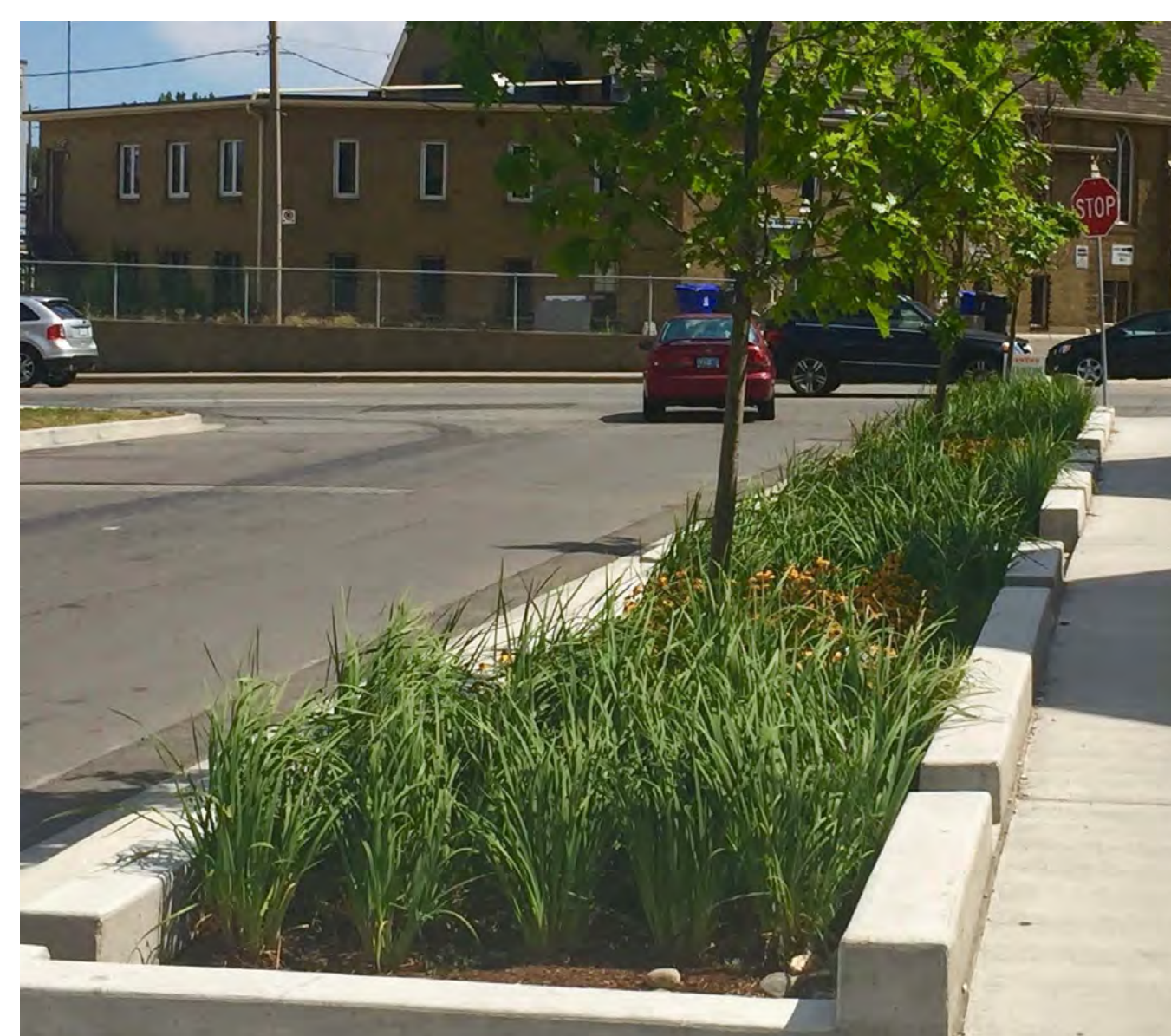
2A Open pit planter with soil cells
