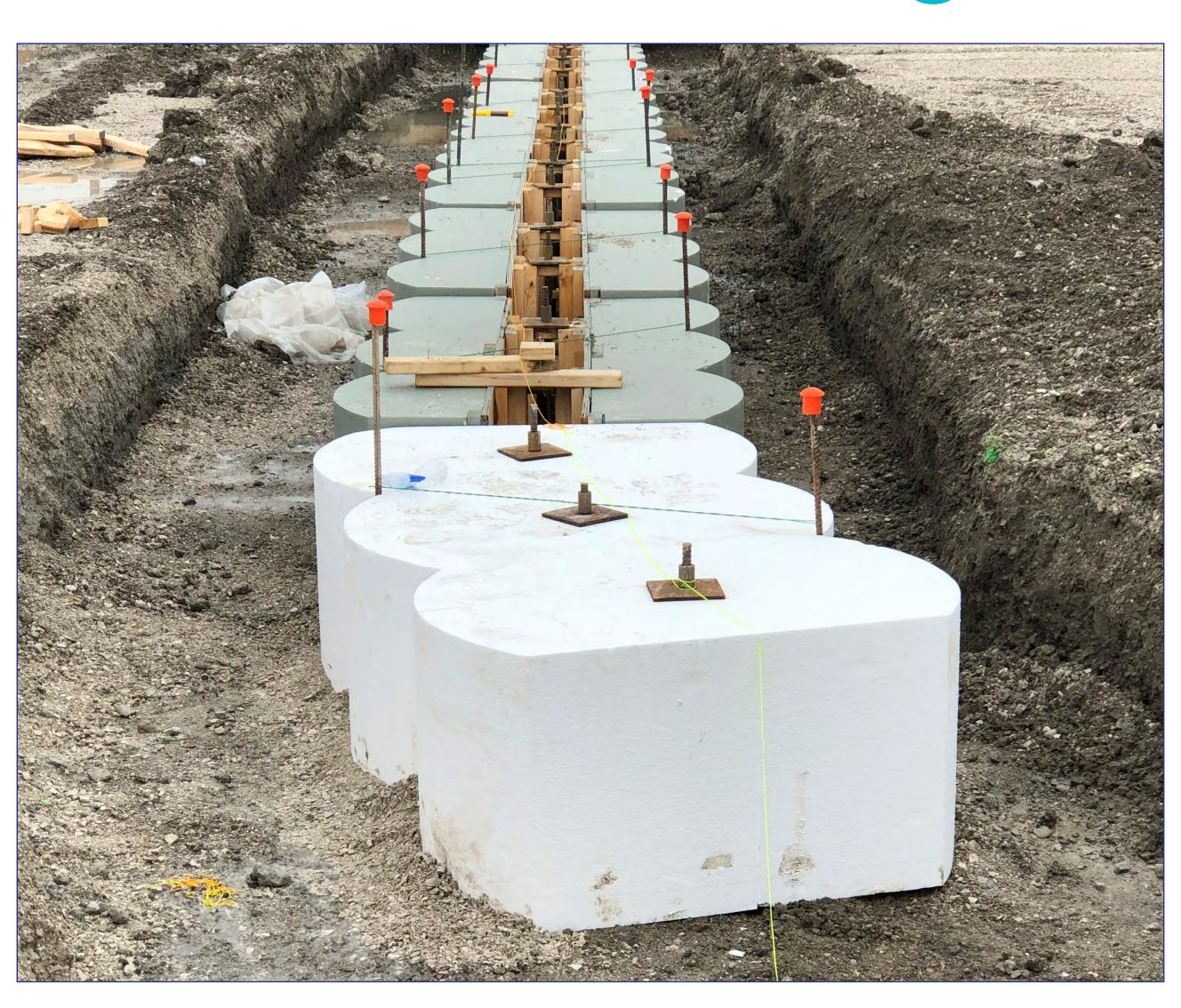
Guide walls line the edges of the new river valley as we prepare to install secant piles for cut-off walls.
