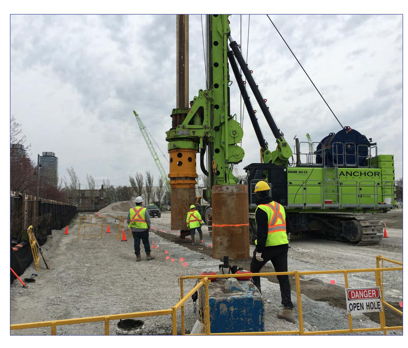
Drill rigs install a secant pile for cut-off walls that will help keep excavation dry and stable.
