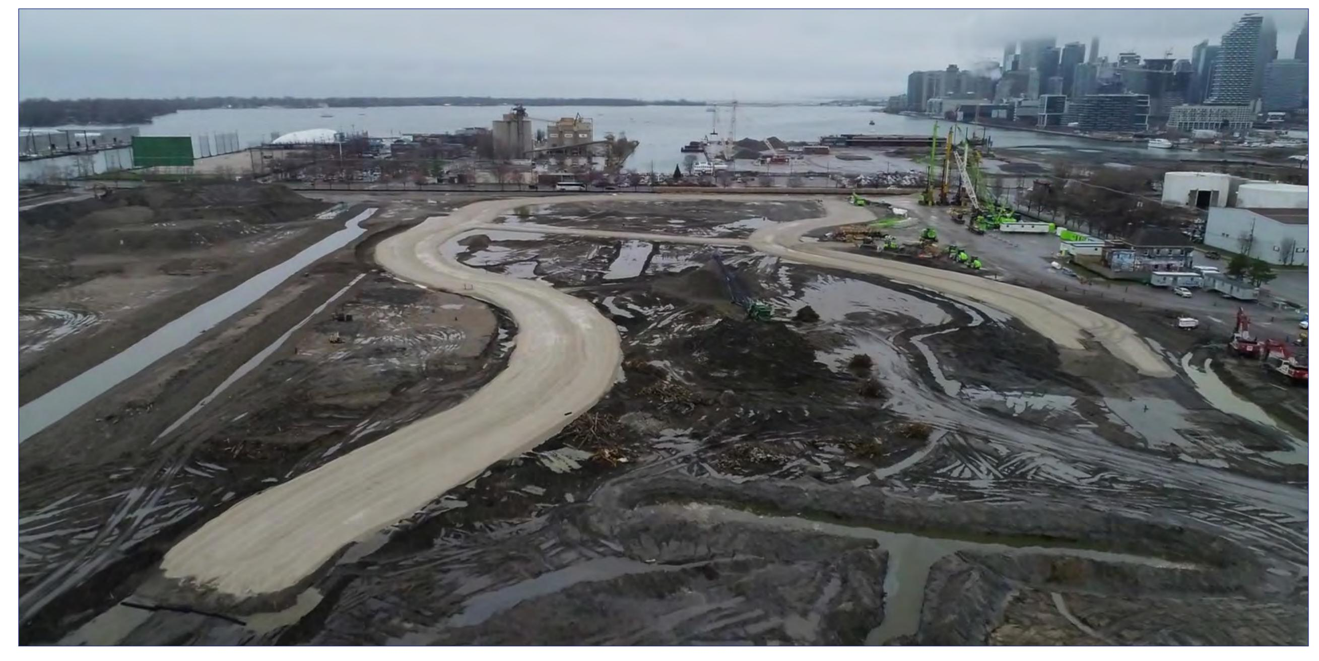
The shape of the first section of the new river valley has been set and crews are ready for deeper excavation.
