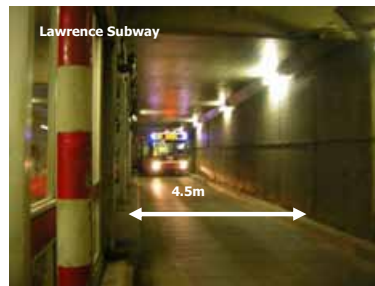
Lawrence Bus Terminal Tunnel
