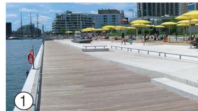
HTO Park East Width: 3m Completion Year: 2007 Wood: Ipe Edge Condition: Galvanized steel toe rail *Underwater
