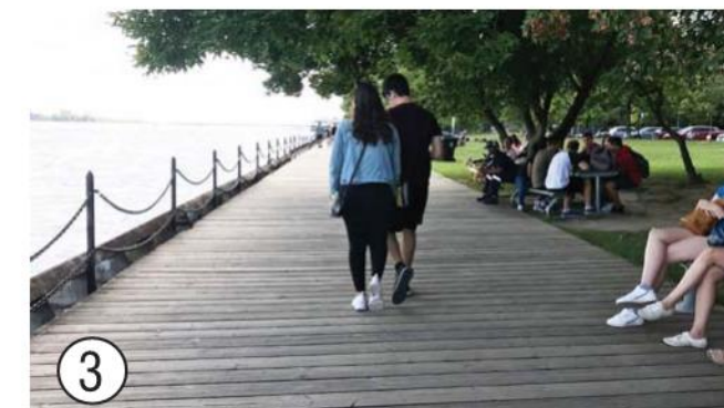
Harbour Square Park East + West Width: 5.3m Completion Year: 1970's, planks replaced in last 7 years Wood: Cedar Edge Condition: Metal Chain Guard Rail
