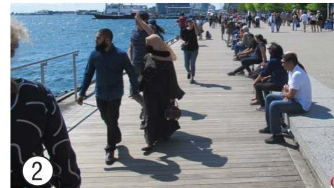
York Quay Boardwalk Width: 5m Completion Year: 2005 Wood: Ipe Edge Condition: Mixed Toe Rail, Guard Rail, Raised Wood Edges
