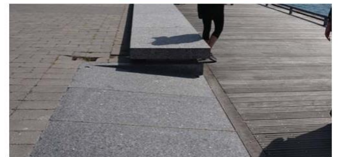
Reference: Granite sloped walkway transition, York Quay
