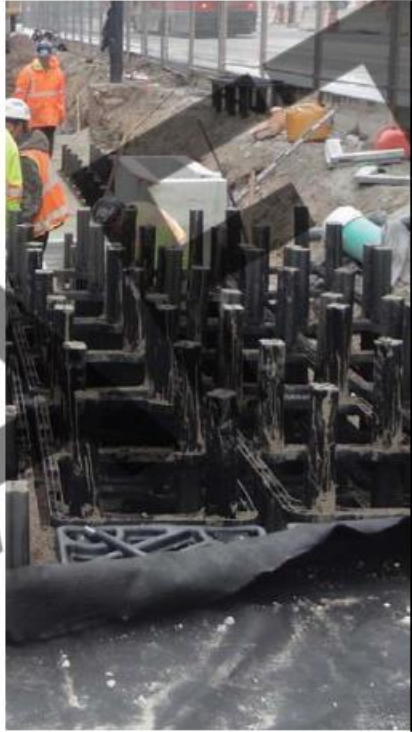
Soil cells to retain water and help tree growth
