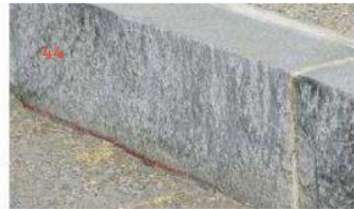
Figure 3.13 Granite curb example
