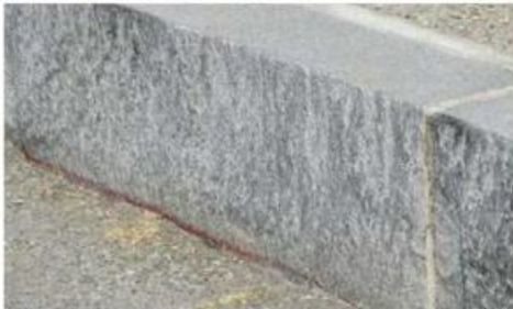
Figure 3.13 Granite curb example
