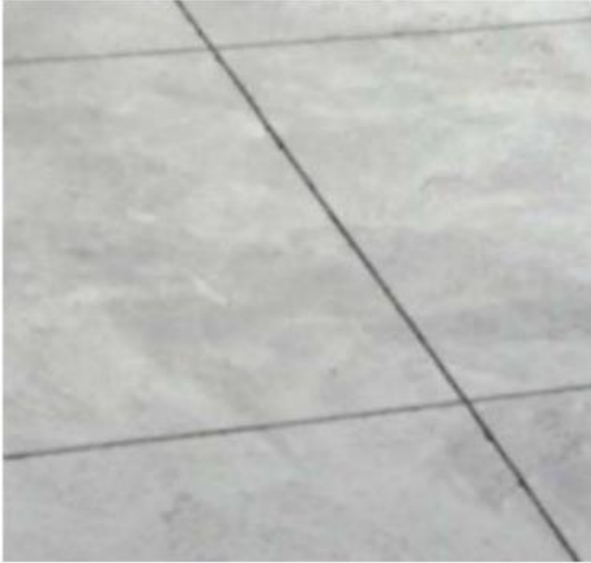
Saw Cut Concrete
