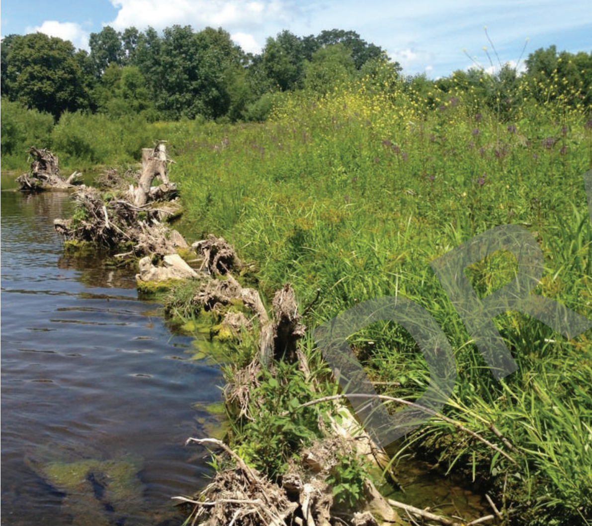
Crib Wall Treatment
