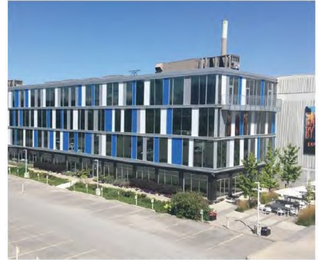
Pinewood Toronto (use of wrapper to activate otherwise blank exterior)
