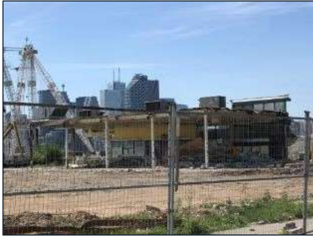
222 Cherry Street – Building demolition ongoing.
