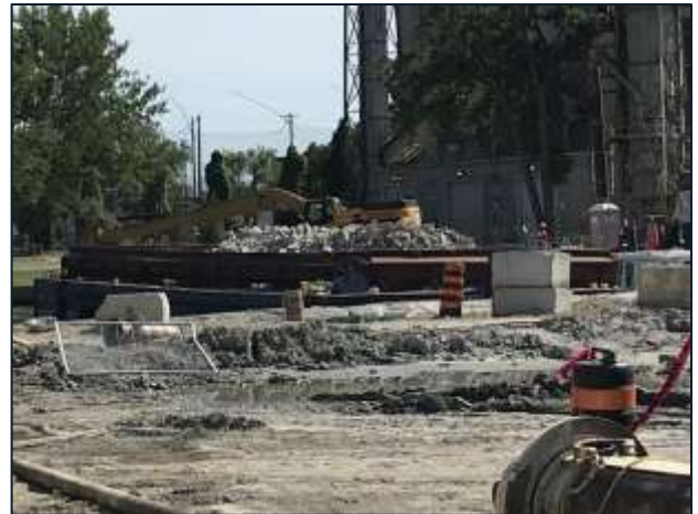
Polson Slip Naturalization – New revetment placement ongoing.
