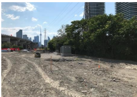
East view transformer install
