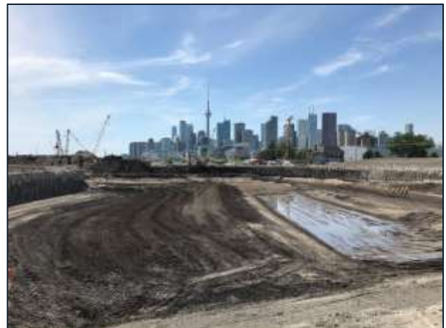
Central River Valley – Final elevation grading operations ongoing.
