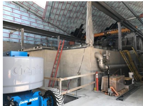
Inside process piping work
