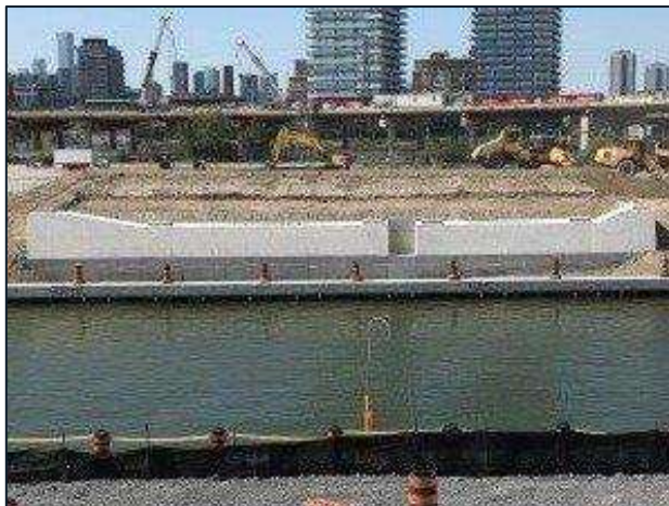
Cherry Street Bridge North – North abutment complete.
