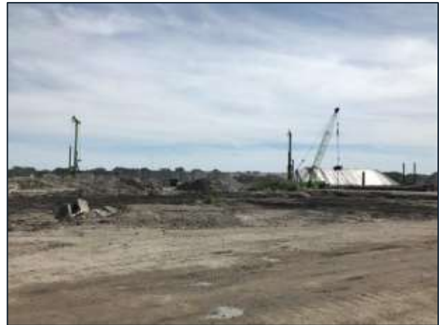
Don Greenway – Spillway shallow excavation ongoing.
