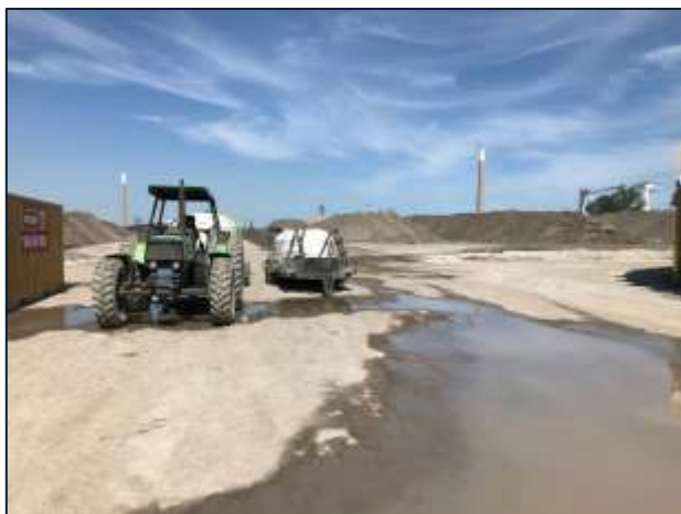
Soil Management & Stockpile – Operations ongoing throughout site.
