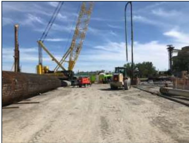
Cherry Street Bridge South – Abutment foundation construction ongoing.
