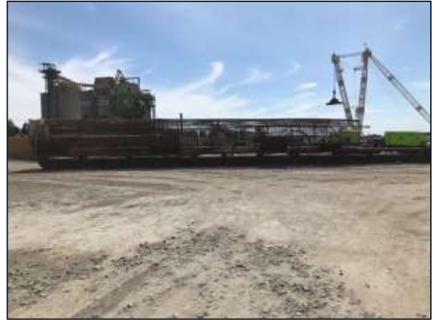
Cherry Street Bridge South – Foundation rebar cages delivered.
