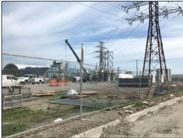
Hydro One Integration – Relocation of towers ongoing.
