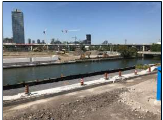
Cherry Street Bridge North – South abutment complete.
