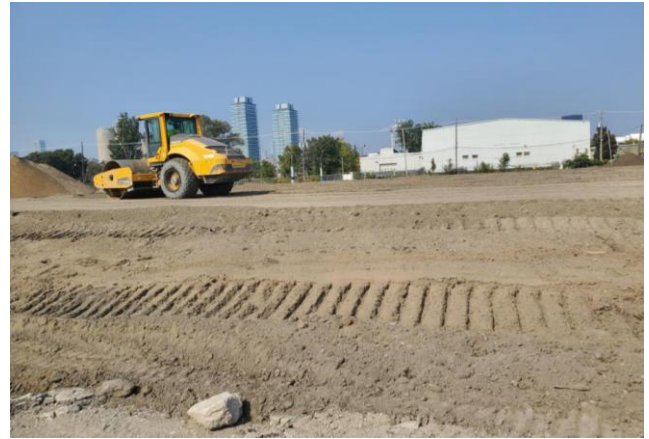
Figure 2 River Park North - Surcharge Installation
