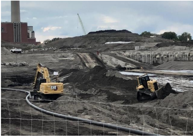
Figure 1 River Valley - Centre Cell Underdrain System Installation
