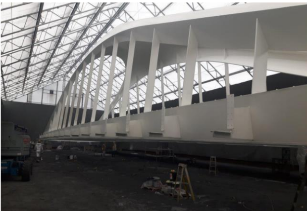
Figure 5 Cherry St Bridge North - Coating Works
