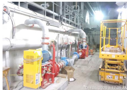
Inside process piping work
