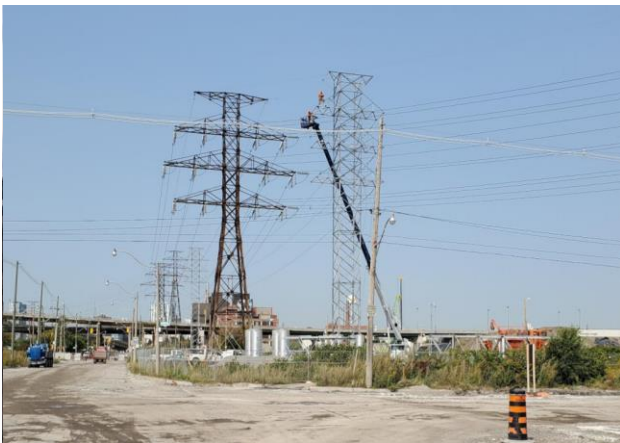
Figure 3 HONI works on Commissioners St/Don Roadway
