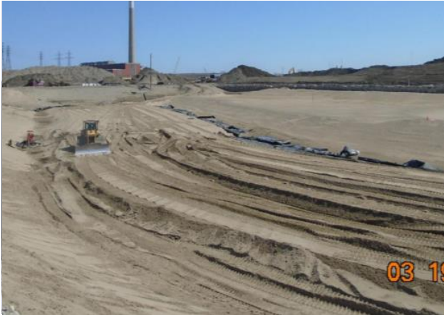
Figure 1 River Valley - Upper 150mm Thick Protective Layer
