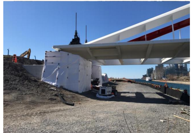
Figure 4 Cherry St North Bridge - Bearings Installation
