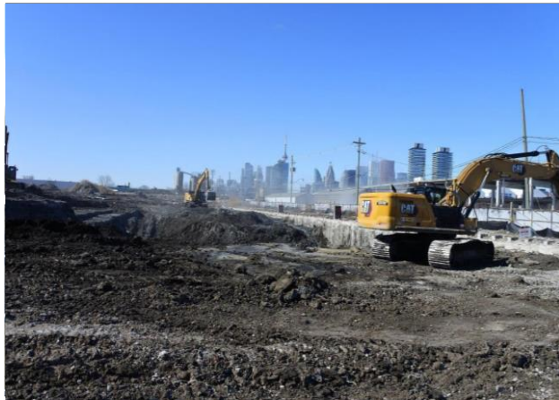
Figure 3 River Valley - Ice Management Deep Excavation
