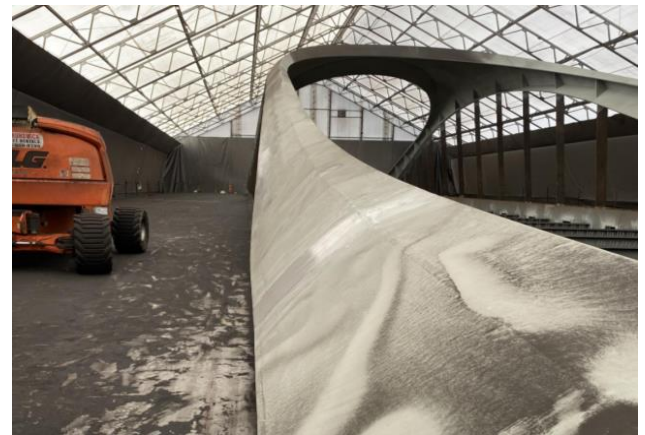
Figure 6 Commissioners St. Bridge (West Half) - Primer Coating
