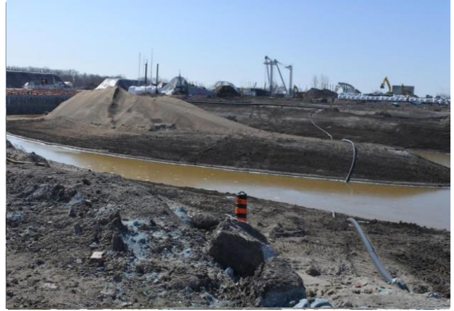
Figure 2 River Valley - Spillway Excavation
