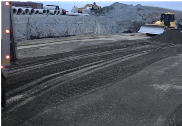
Figure 5 Commissioners St Bridge - Haul Road
