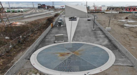
West View and Storm Shaft
