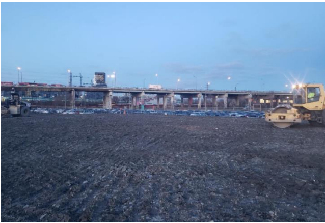
Figure 3 Cherry St Backfilling (3C Area)
