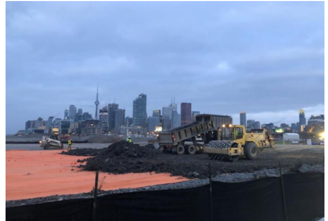
Figure 4 Cherry St Backfilling/Surcharging South of Keating Channel
