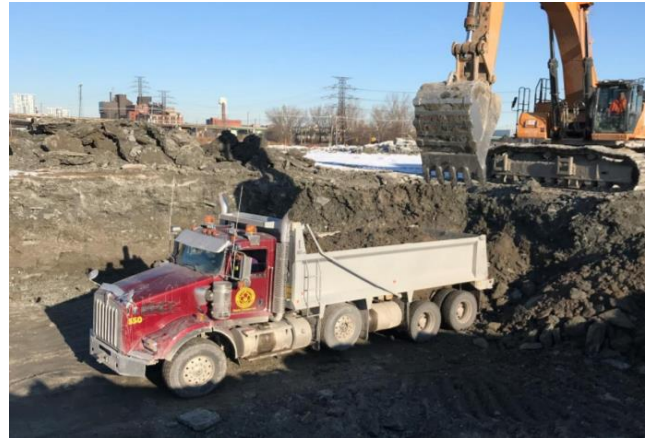
Figure 2 Shallow Excavation South of Commissioners St
