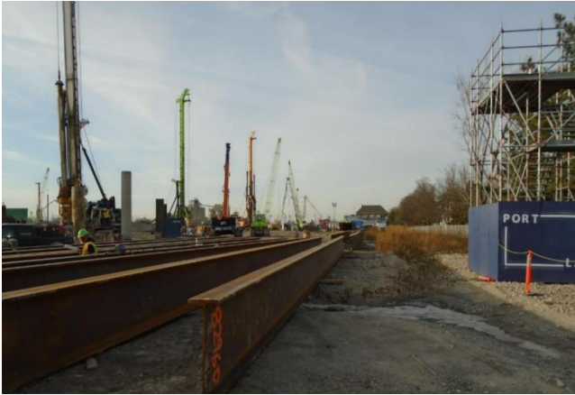
Figure 1 River Valley System Cut Off Walls
