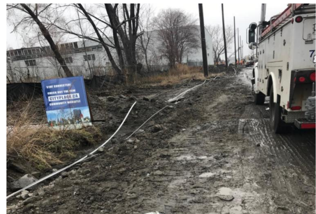
Figure 6 Commissioners St - Utilities Removal
