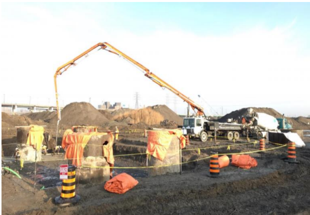
Figure 5 Commissioners St Bridge - Foundation Works
