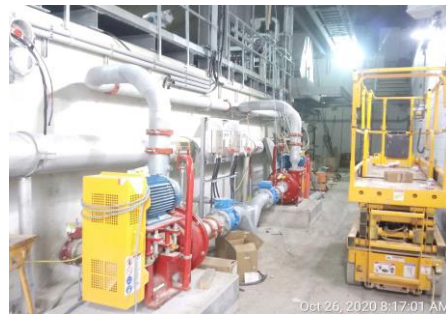
Inside process piping work
