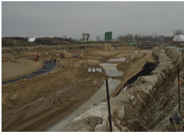
Figure 3 River Valley - Backfill Along Cut-off Wall
