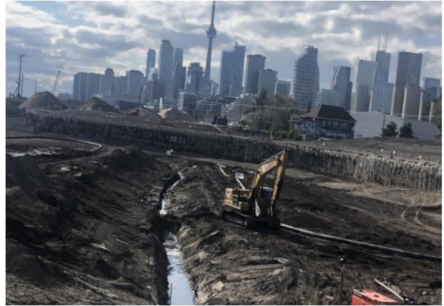
Figure 2 River Valley - Under Drain Installation
