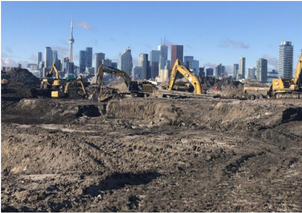
Figure 1 River Valley - Spillway Deep Excavation
