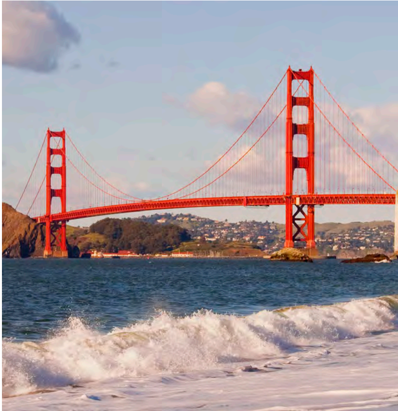
Golden Gate Bridge
