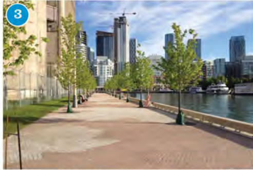
3 Portland Slip Promenade Phase I Size: 0.12 hectares (0.29 acres) Budget: $2.5 million Design Oversight: Waterfront Toronto Landowner: City of Toronto Approvals Process: Parks Department Approval Funding Sources: Waterfront Toronto Tripartite Construction Oversight: Waterfront Toronto O&M Lead: City of Toronto Date of Completion: June 2014
