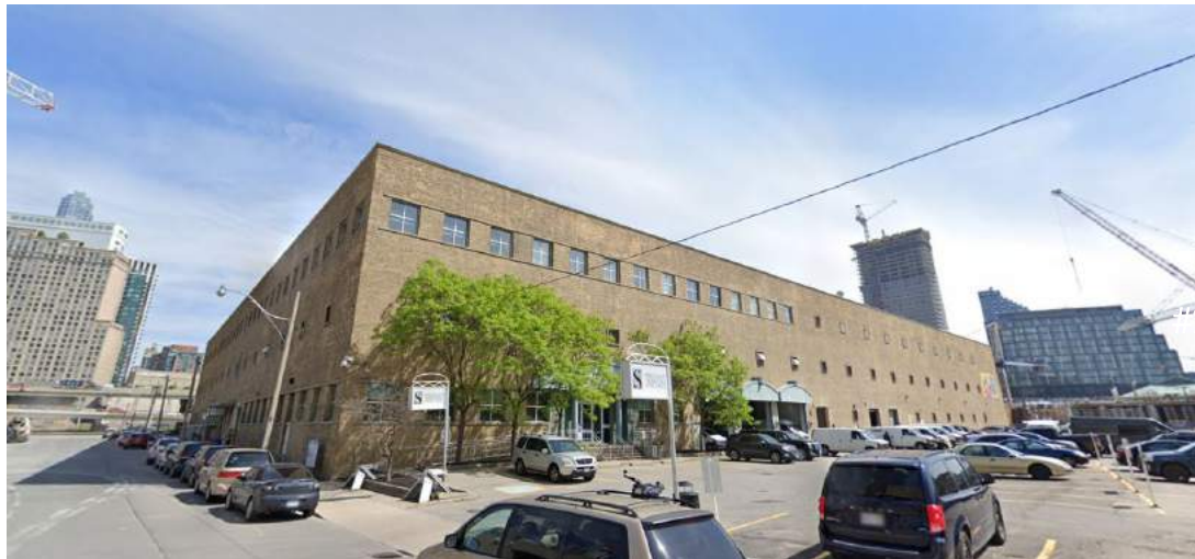
Looking northeast from Freeland St.
