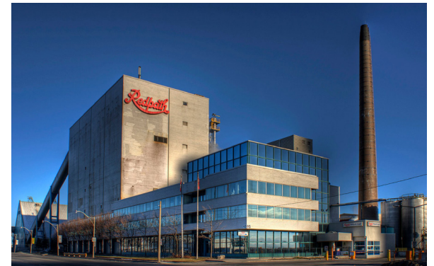
Figure 2.5 - Redpath Sugar Facility
