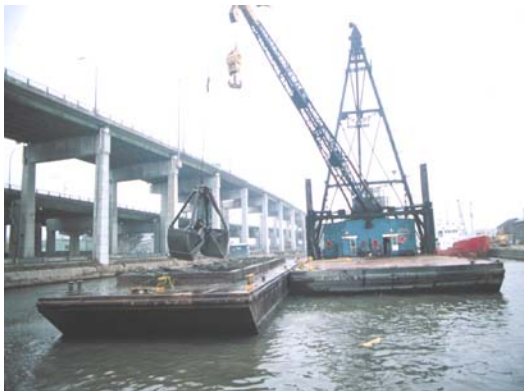
Ongoing Dredging the Keating Channel
