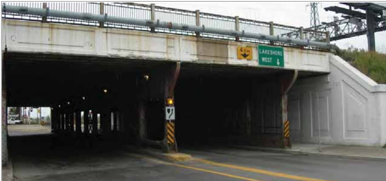
Figure 6-1 Cherry Street Underpass of Rail Corridor
