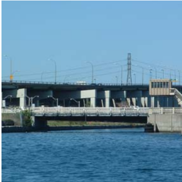
EXISTING CHERRY STREET BRIDGE
