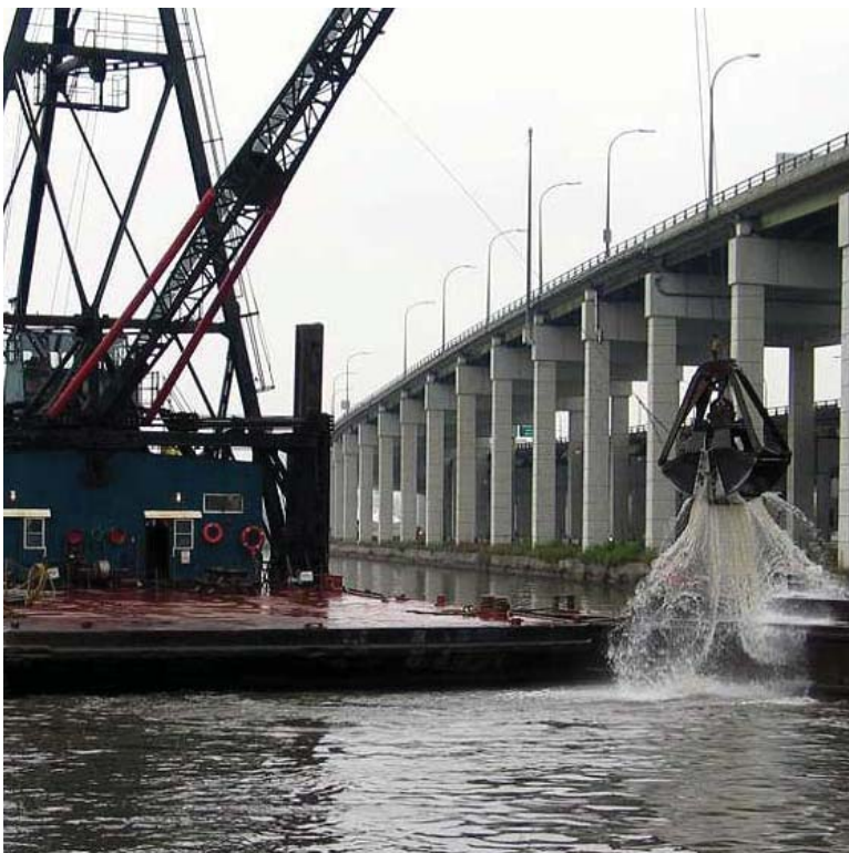
DREDGING ON THE KEATING CHANNEL
