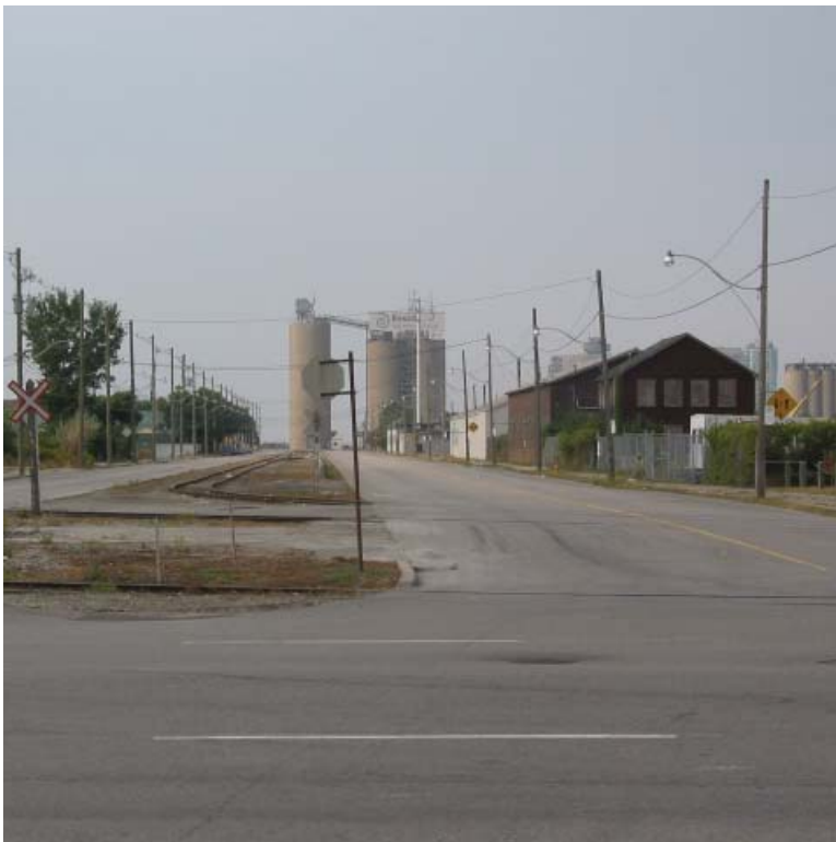
VILLIERS STREET LOOKING WEST TOWARDS ESSROC PIER
