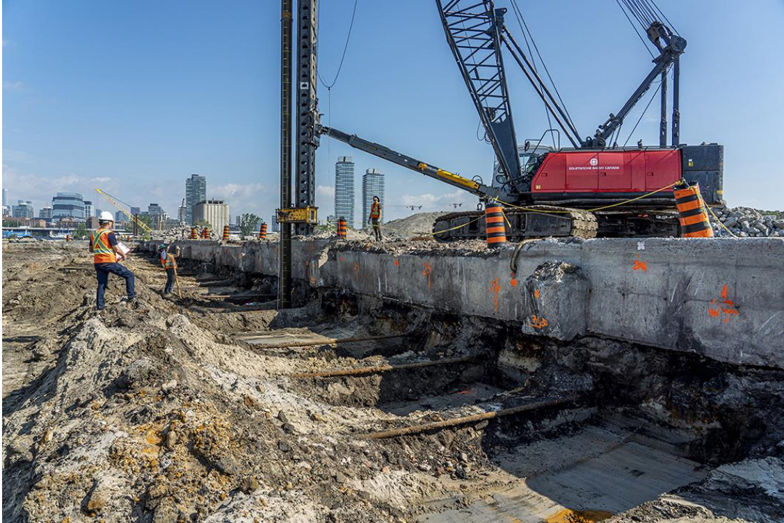
Above: To reinforce the dockwall where the Marine Terminal 35 building used to be, crews first had to expose the existing tie-backs (the metal rods shown here), before installing new ones.
