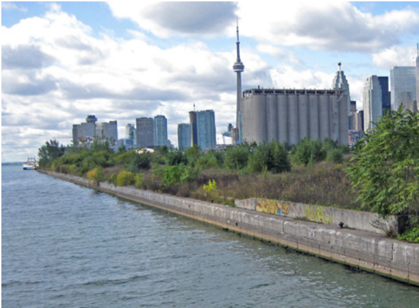
Figure 28 Keating Channel and Existing Concrete Dockwall with Timber Sheetpile
