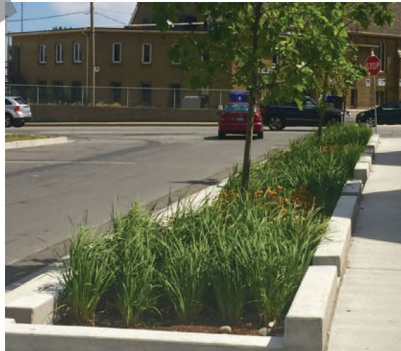
2A Open pit planter with soil cells
