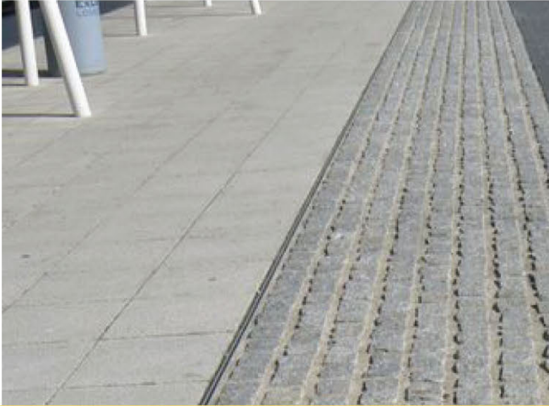
Concrete Pavement with Granite Buffer
