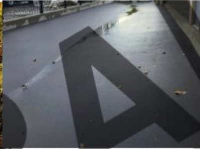
Solar Reflective Coating
