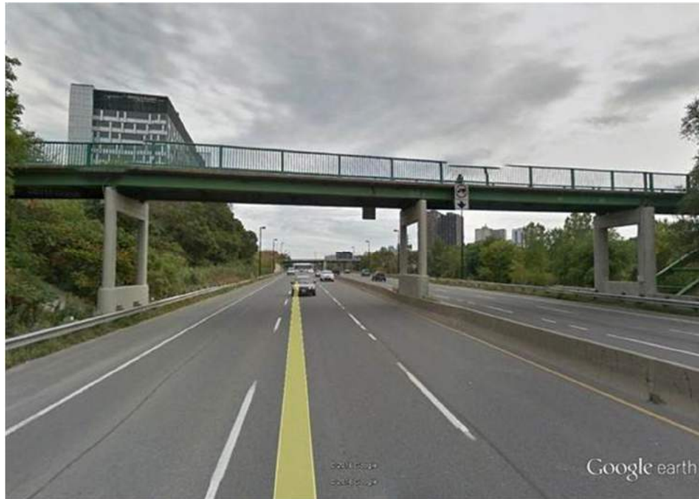
Example of Grounded Bridge - Riverdale Park Pedestrian Bridge, Toronto, ON
