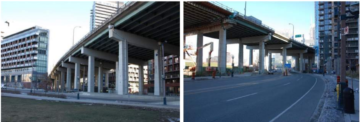
Photos of elevated Gardiner Expressway over Fort York Boulevard (looking east).
