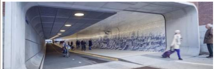
Cuyperspassage, pedestrian and cycling tunnel, Amsterdam, Netherlands
