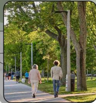
DIRECT BURY CONCRETE LIGHT POSTS
