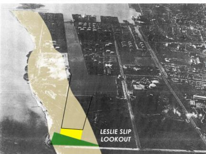
1949 FISHERMAN'S ISLAND BAR BEFORE BACKFILLING CLAUDE CORMIER + ASSOCIÉS INC
