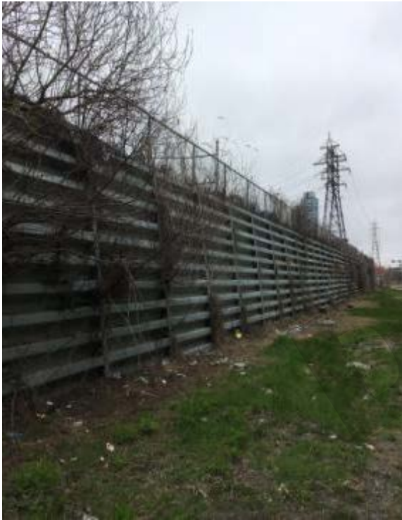
Existing Bin Wall
