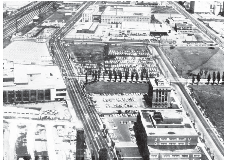
Historical view of the Lake Shore Boulevard looking east from York Street (1950s)(source: Toronto Archives)
