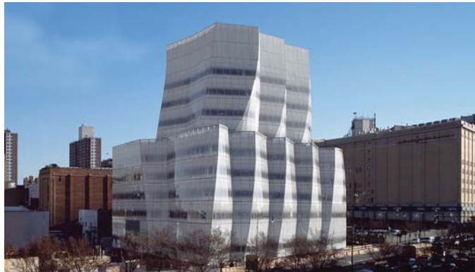
IAC Building, New York, USA 3
