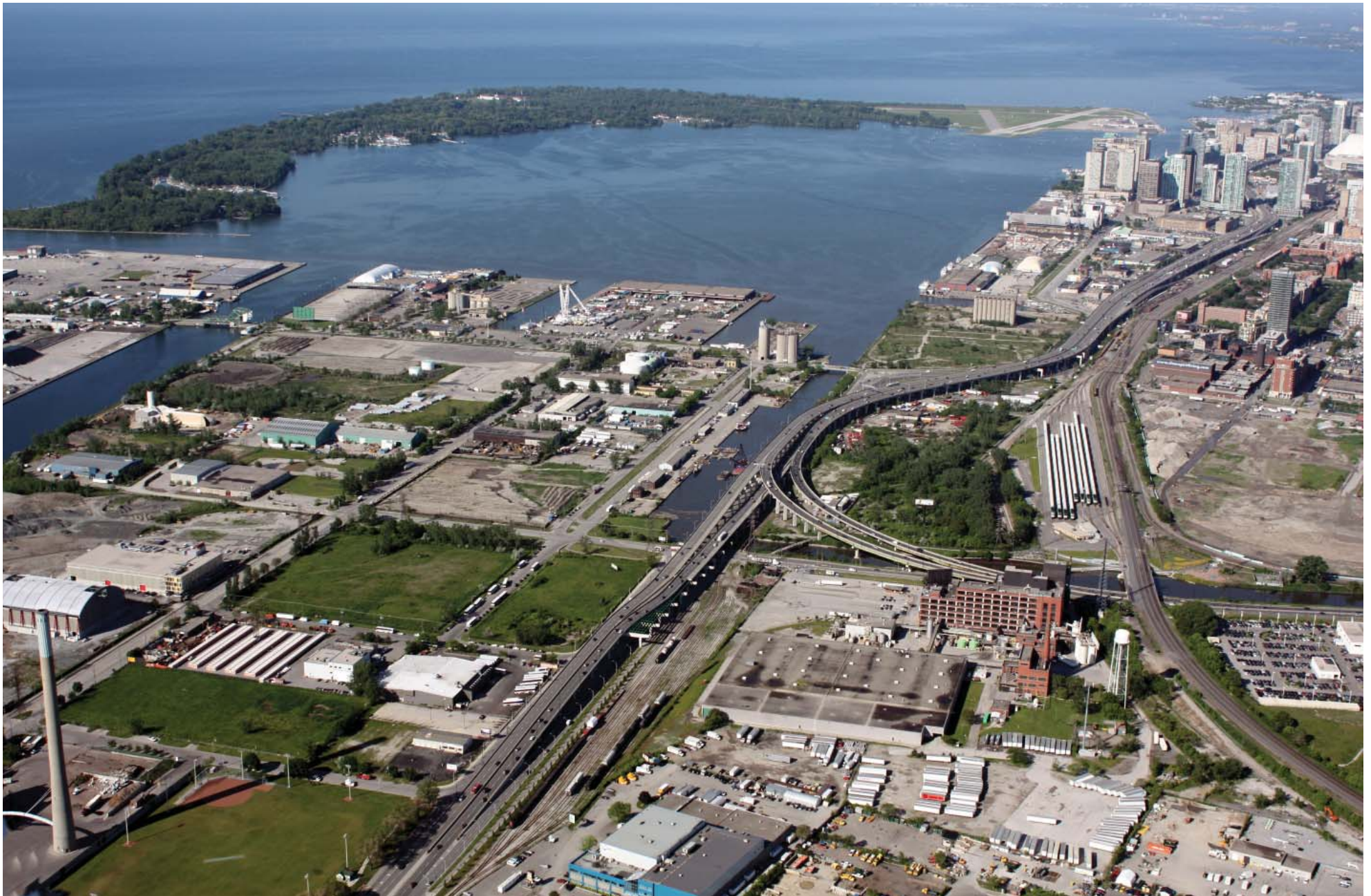
View of the Gardiner Expressway and Lake Shore Boulevard Corridor looking south-west from the Port Lands.
