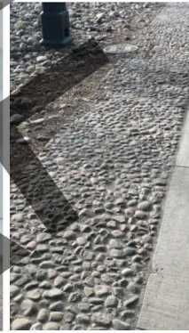
Stabilized stone as median edge
