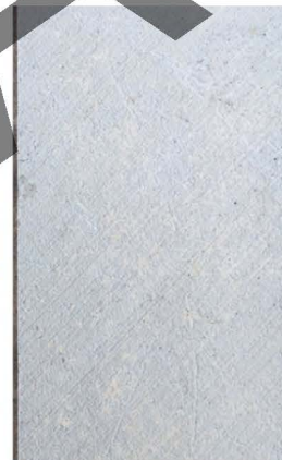
BROOM FINISH ONE DIRECTION (CITY OF TORONTO STANDARD)
