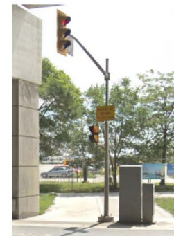
Ensure all poles are straight and aligned with intersections, not obstructing circulation pathways and waiting zones
