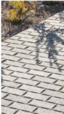
Permeable concrete unit pavers
