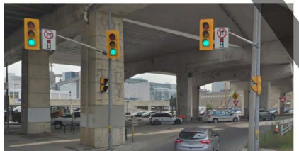
Duplicate traffic lights and signs
