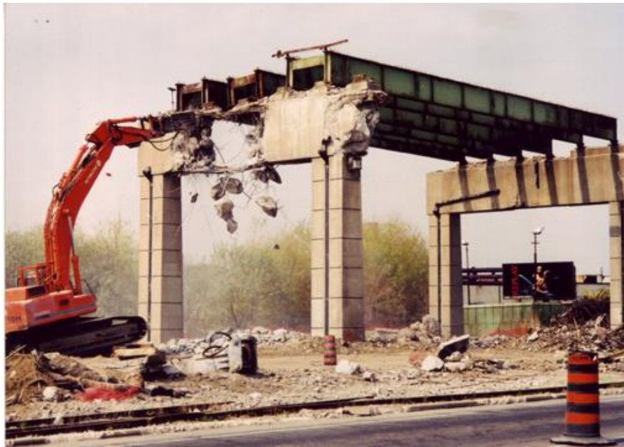
Figure 6-2: Gardiner Deck Removal (2001) East of Logan Avenue
