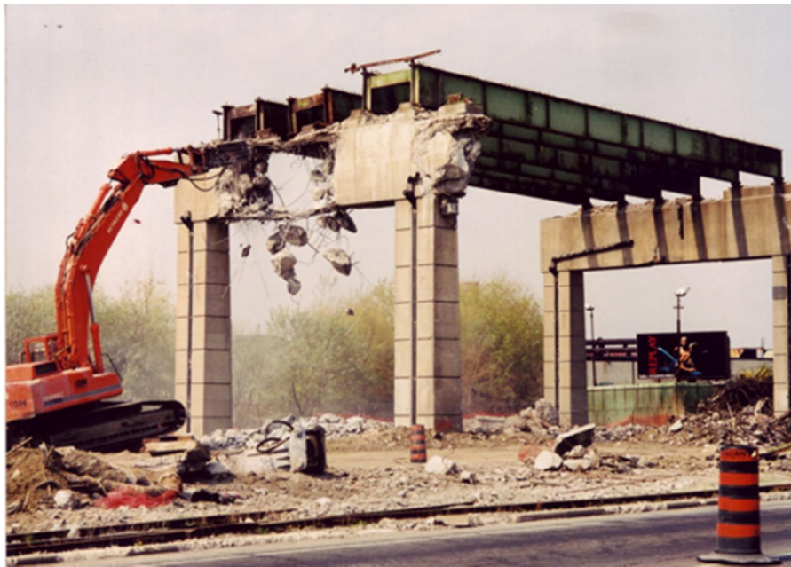
Figure 6-2: Gardiner Deck Removal (2001) East of Logan Avenue
