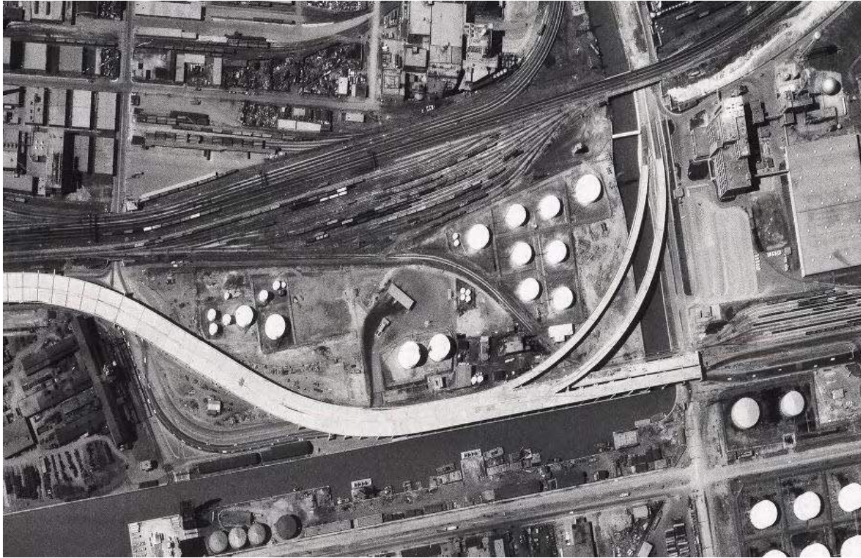
Figure 3.8: 1964 Aerial Photograph of Keating Channel Precinct Area
