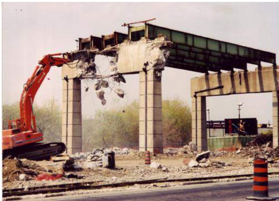
Figure 6.2: Gardiner Deck Removal (2001) East of Logan Avenue
