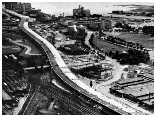
1958: Building of the Gardiner Expressway, routed through industrial waterfront.
