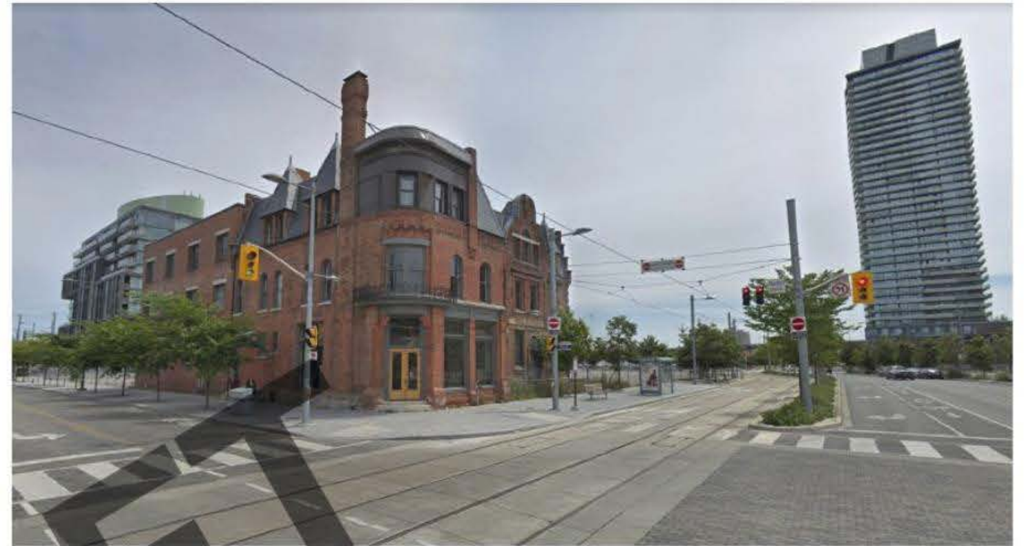
VIEW FROM CHERRY AND FRONT STREET LOOKING SOUTHEAST
