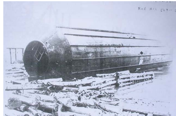
Figure A 4: The Roller Boat undergoing renovations, possibly those of 1902. Note the exterior paddles had been extended along the entire length of the hull, although by 1902 the roller function was abandoned.
