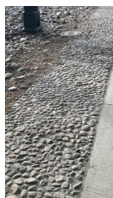
Stabilizing stone as median edge
