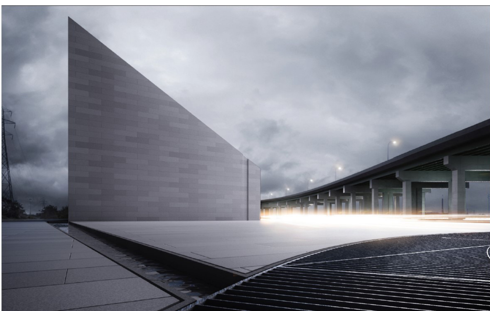
Rendering of the Cherry Street Stormwater Facility from the storage shaft
